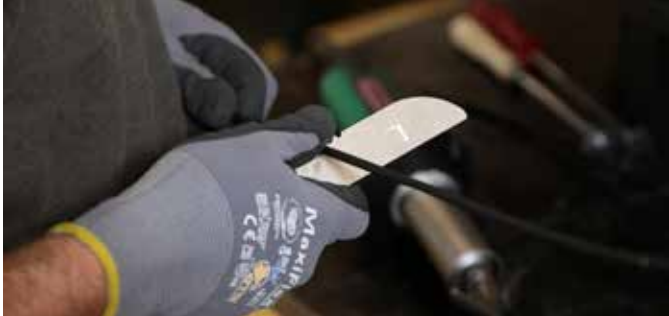
Remove the oxide layer from the welding rod.
