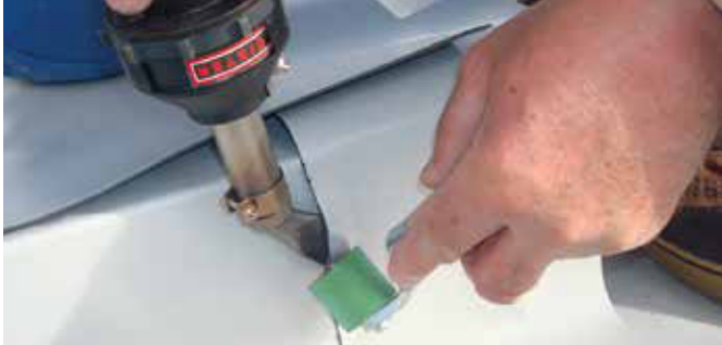
HOT JET S with angled nozzle welding a T-joint on the roof.
